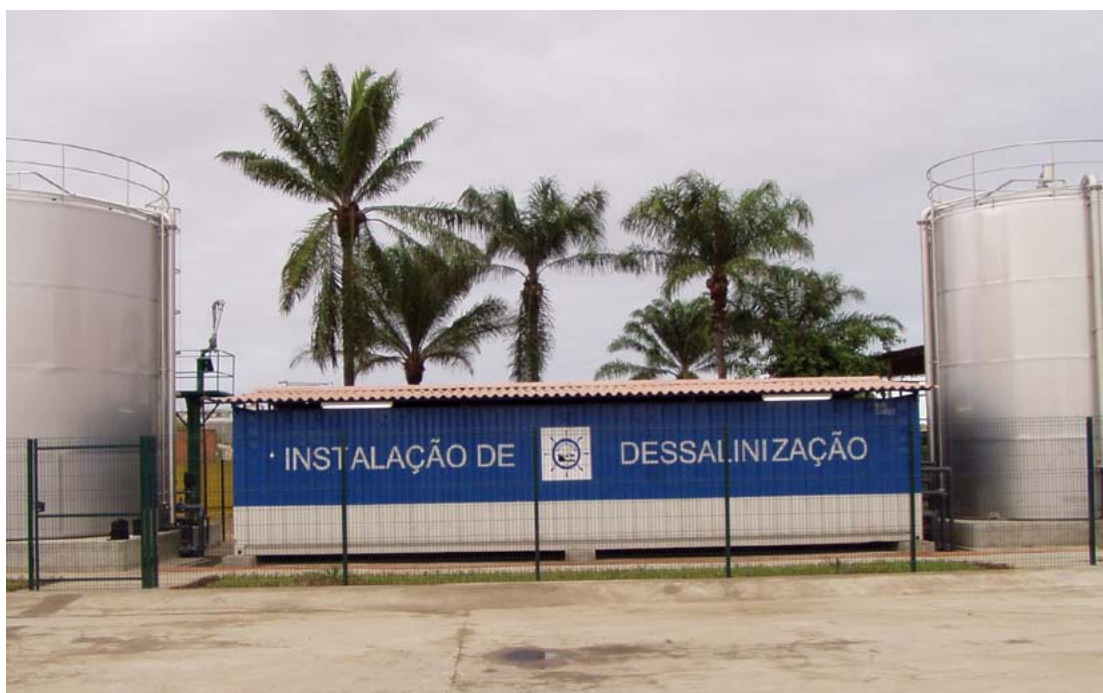
Reverse osmosis desalination plant Gefico installed in container.
