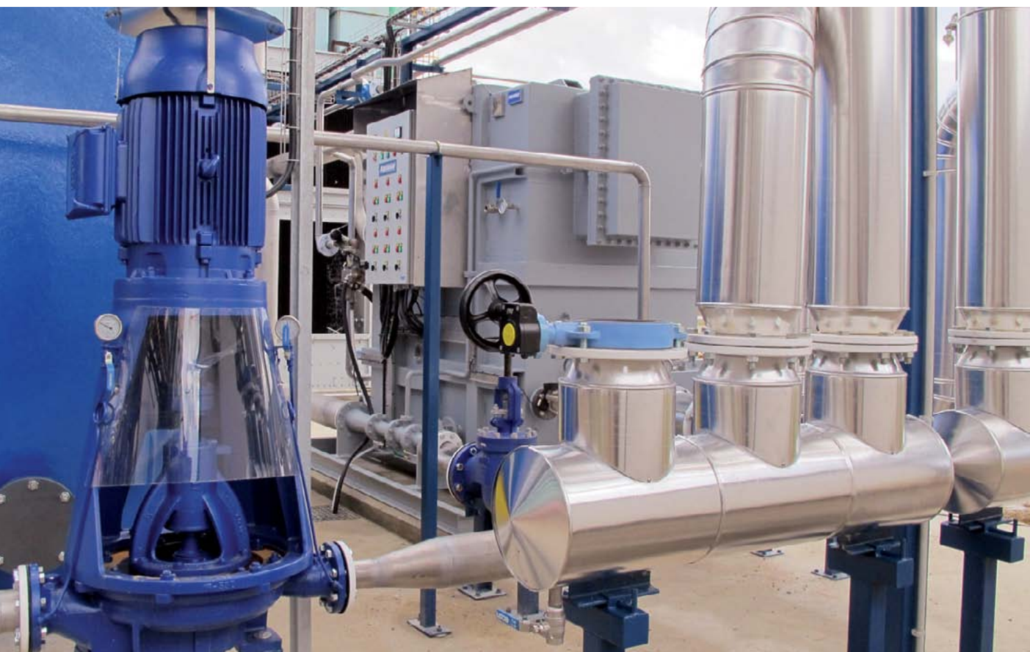
Power plant, equipped with 1 fresh water generator GEFICO Evaporator model AQ-100/120A. Viscofan Group. Spain.
