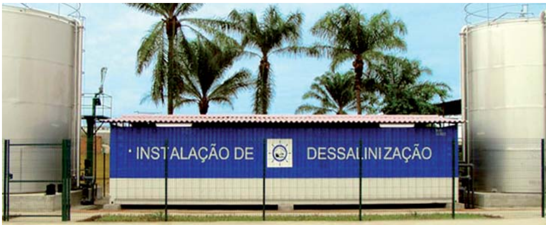
Two reverse osmosis units Gefico, model AQE-60D, in two 40 feet container with pre and post-treatment to obtain drinking water. Porto do Lobito - Angola.
